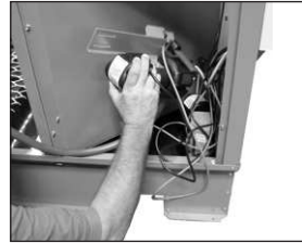
Remove the entire pump/chlorinator assembly
