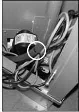
Cut the cable tie
